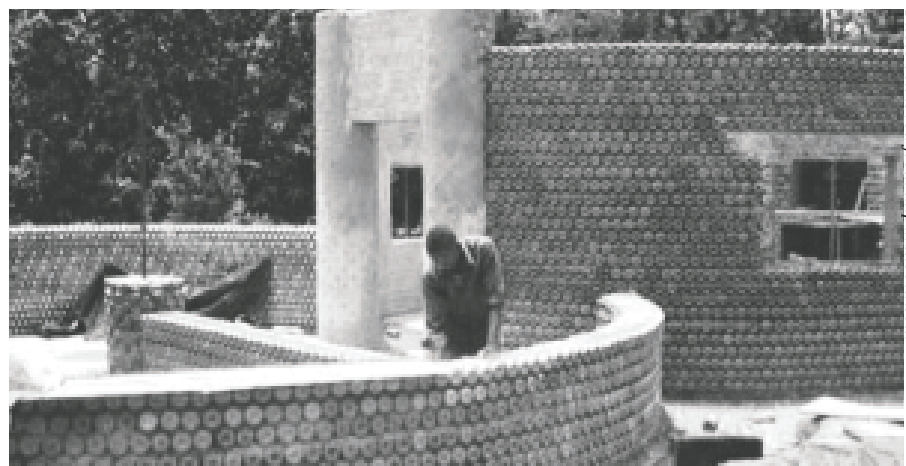
A building made of water bottles in Nigeria.
