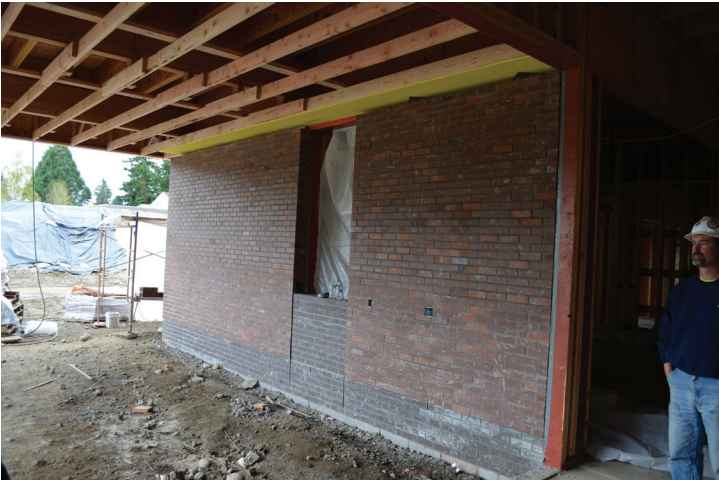
Work has already begun on installing the brick exterior of the building.
