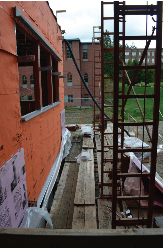
Scaffolding along the south wall allows workers to continue laying the brick exterior.
