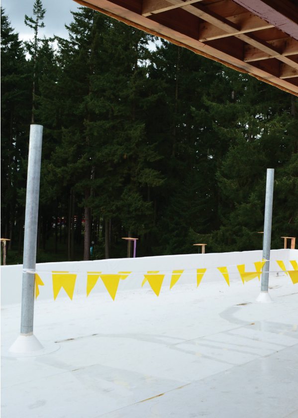
When the building is finished, these poles will hold an interactive solar panel system where engineering students can get hands-on experience with solar power and the effects of sunlight angles on energy production.
